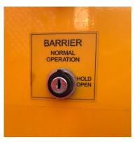
are interrupted before the barrier closes, it will return to the upright, open position and re-set the wait time delay before trying to close once again. The barrier will not respond to the fob while being held open by this control.
